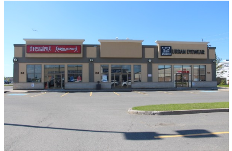
UNIT C1A: 1,007 Square Feet
